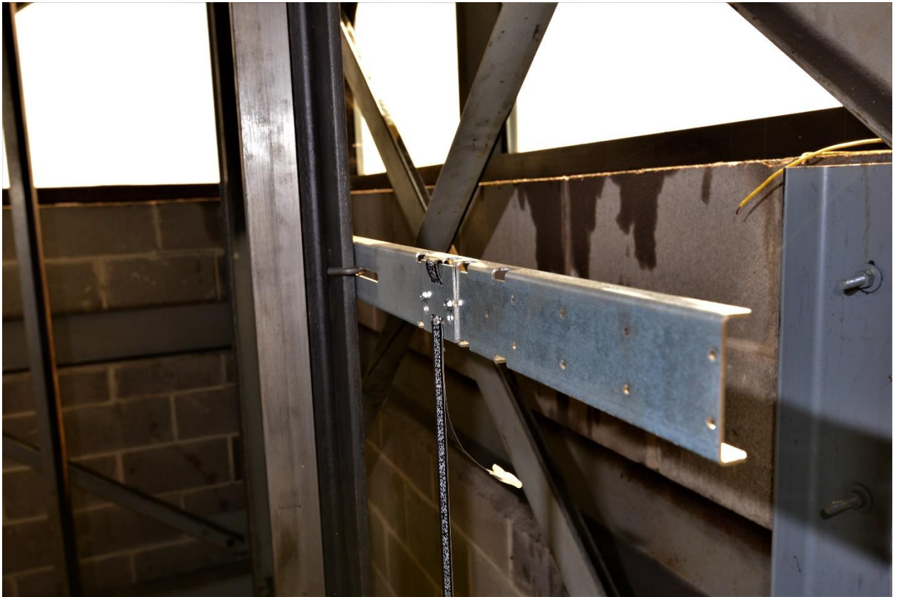
Figure E1.1: Top Tape Bracket
